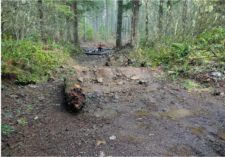
Berm on temporary road accessing North Units 16 and 18
