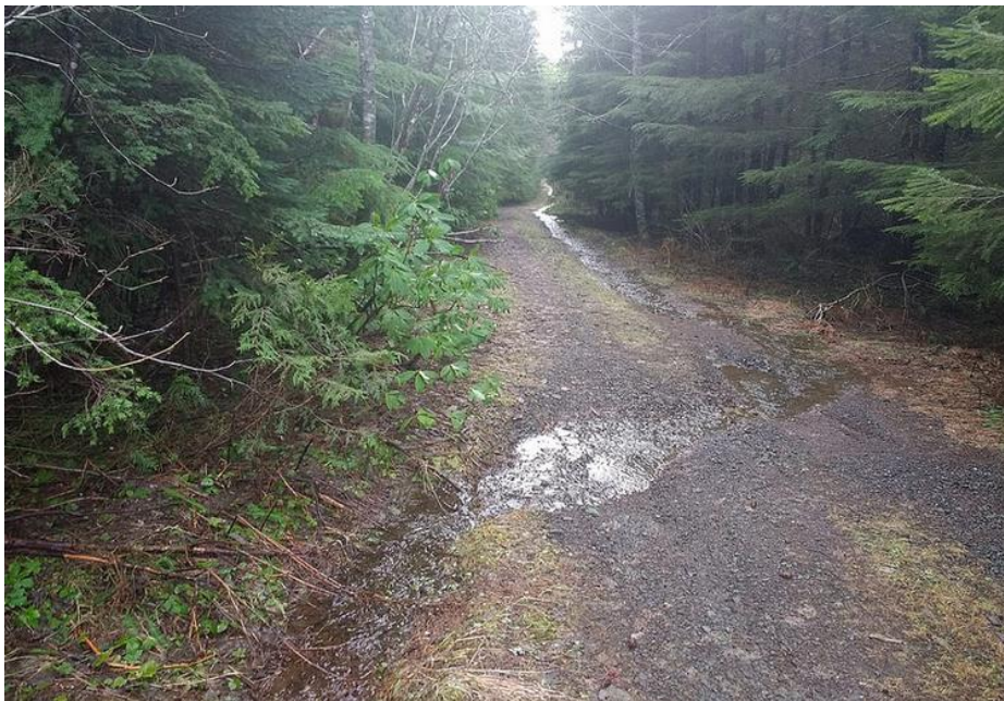
Gully erosion at junction of 4614-150 and 4614-160 (above and below)
