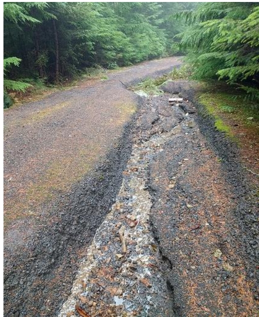
Uncontrolled gully erosion on 4613 near Whisky Creek and adjacent to Unit 176 (above), and on 4613-140 (below)
