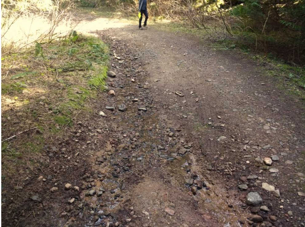
Water-filled gully which runs down the 4610-153 road and terminates at stream crossing, fed by seep at 45.21958, -122.09056
