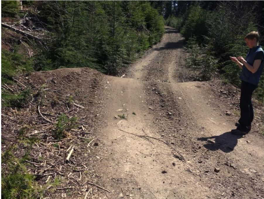
Berm on 4610-155 shortly after it enters North Clack Unit 342
