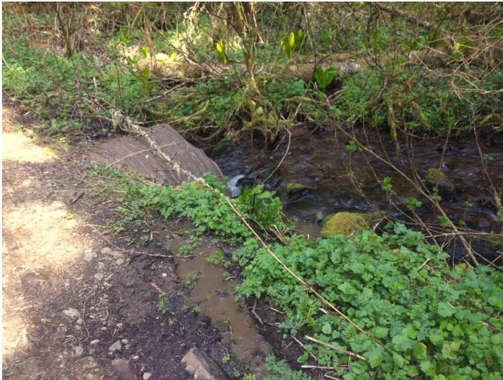
4614-120 Whiskey Creek crossing, road sediment entering stream
