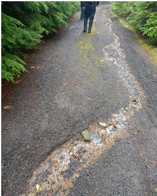
Uncontrolled gully erosion on 4613 near Whisky Creek and adjacent to Unit 176 (above), and on 4613-140 (below)
