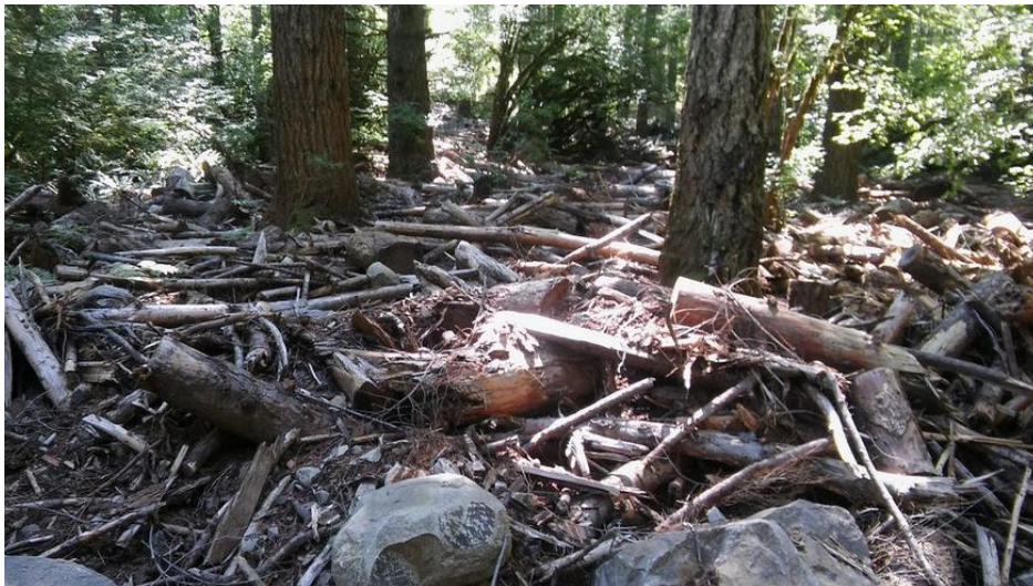
Deep slash and boulder placement to deter illegal OHV use in damaged areas adjacent to the 4610 road
