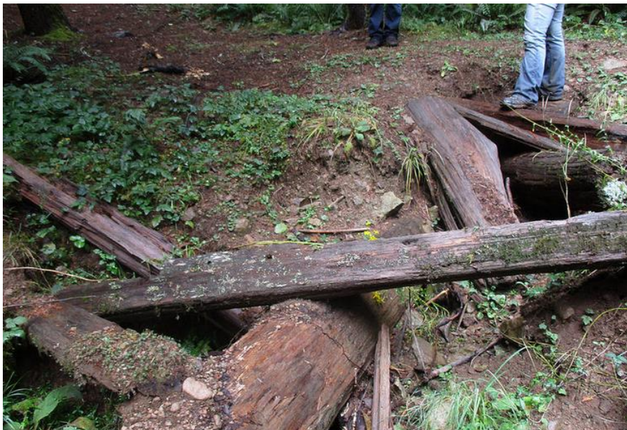
FSR 4613-016 muddy road conditions (above) leading to deteriorating stream crossing at Whisky Creek tributary (below)
