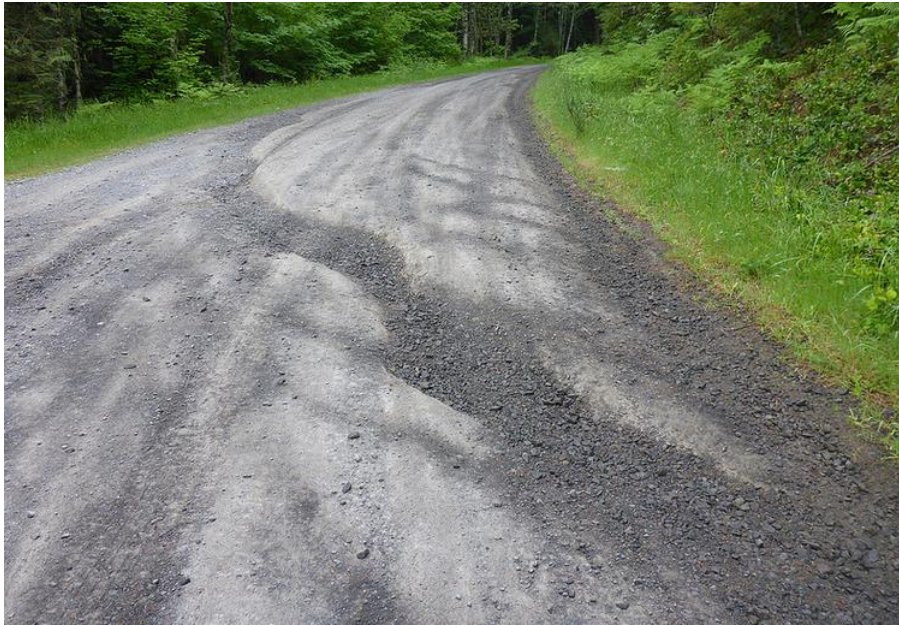
Uncontrolled gully erosion on 4613 near Whisky Creek and adjacent to Unit 176 (above), and on 4613-140 (below)
