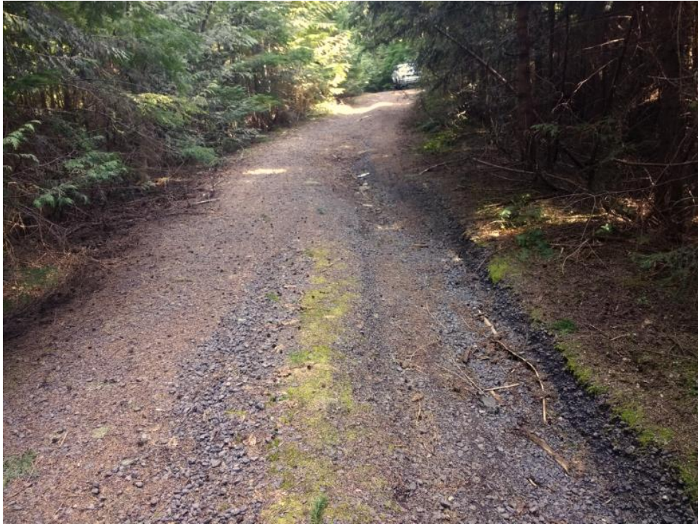
Gully erosion along the 4613-130 road at 45.22937, -122.12789
