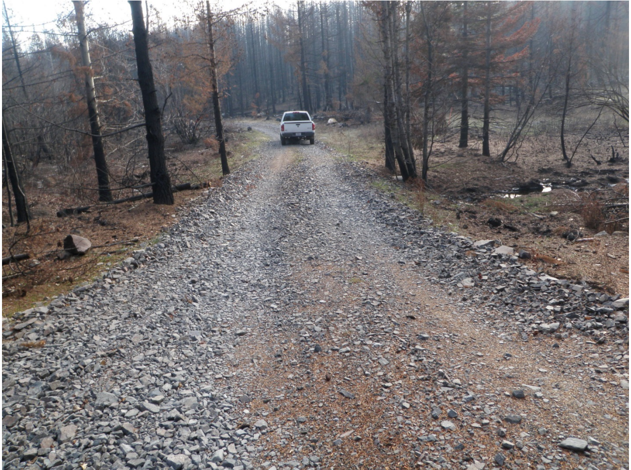
Figure 3-16: Photo showing the 1711 road crossing of Mosier Creek. The crossing is flat and well rocked.
