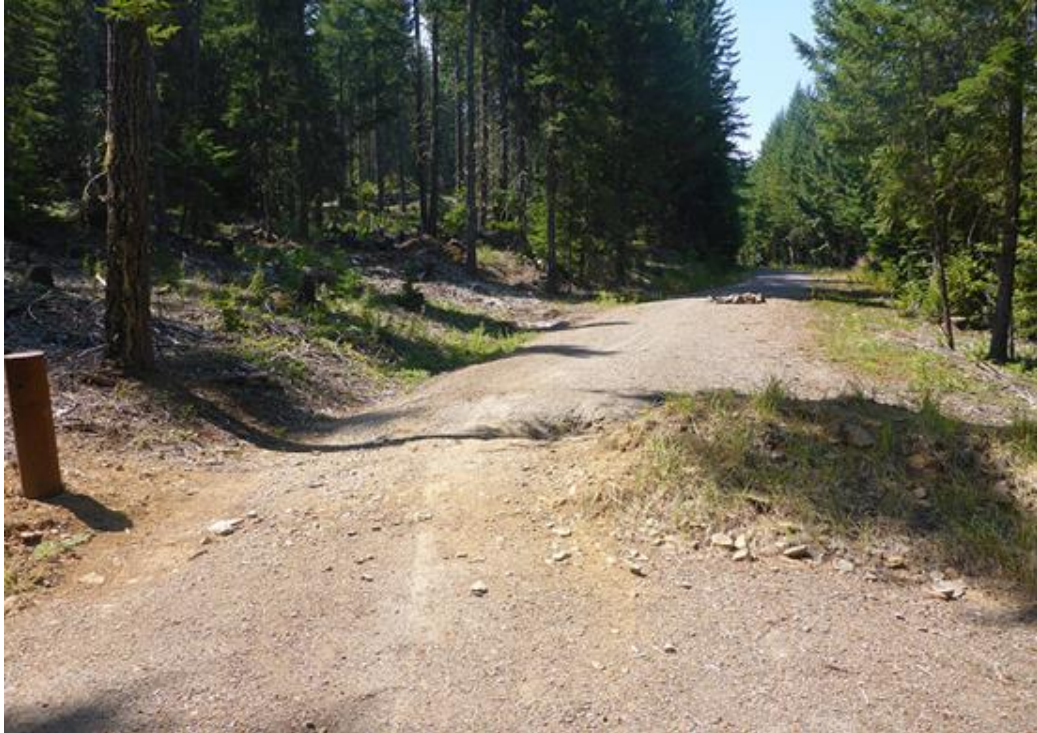
Figure 5: Breached berm on closed road 4660-140 (closed with Increment 2) in the Hunter project area
