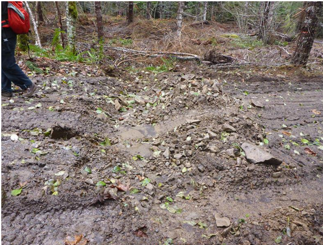
Figure 4: Road 6311-130 reopened as part of the Jazz Thin, unregulated access damaging erosion control measures
