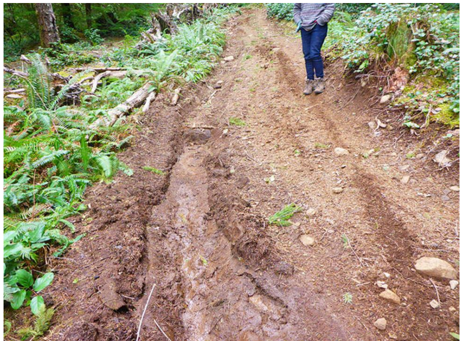
Figure 2: OHV damage at Goat Mtn Unit 38, which includes additional roadbuilding
