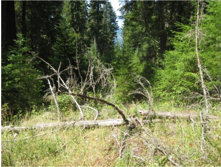
Figure 2-4: Example of a Decommissioned Road
