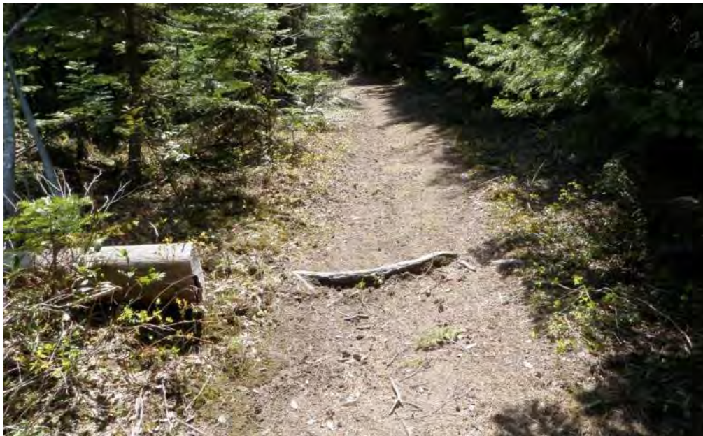
Figure 38. Photograph of a portion of the proposed temporary road accessing blocks 4 and 7 that is within a Riparian Reserve. The road is currently open and being used as a trail.
