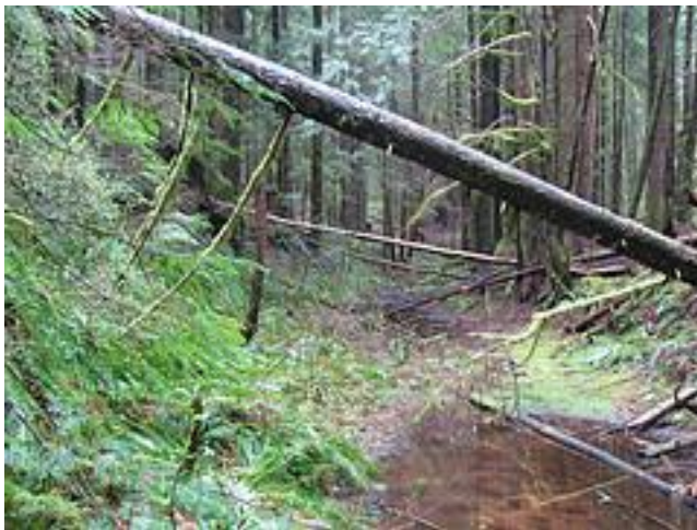
Trees falling and water pooling in the “road” 1N-5E-36
