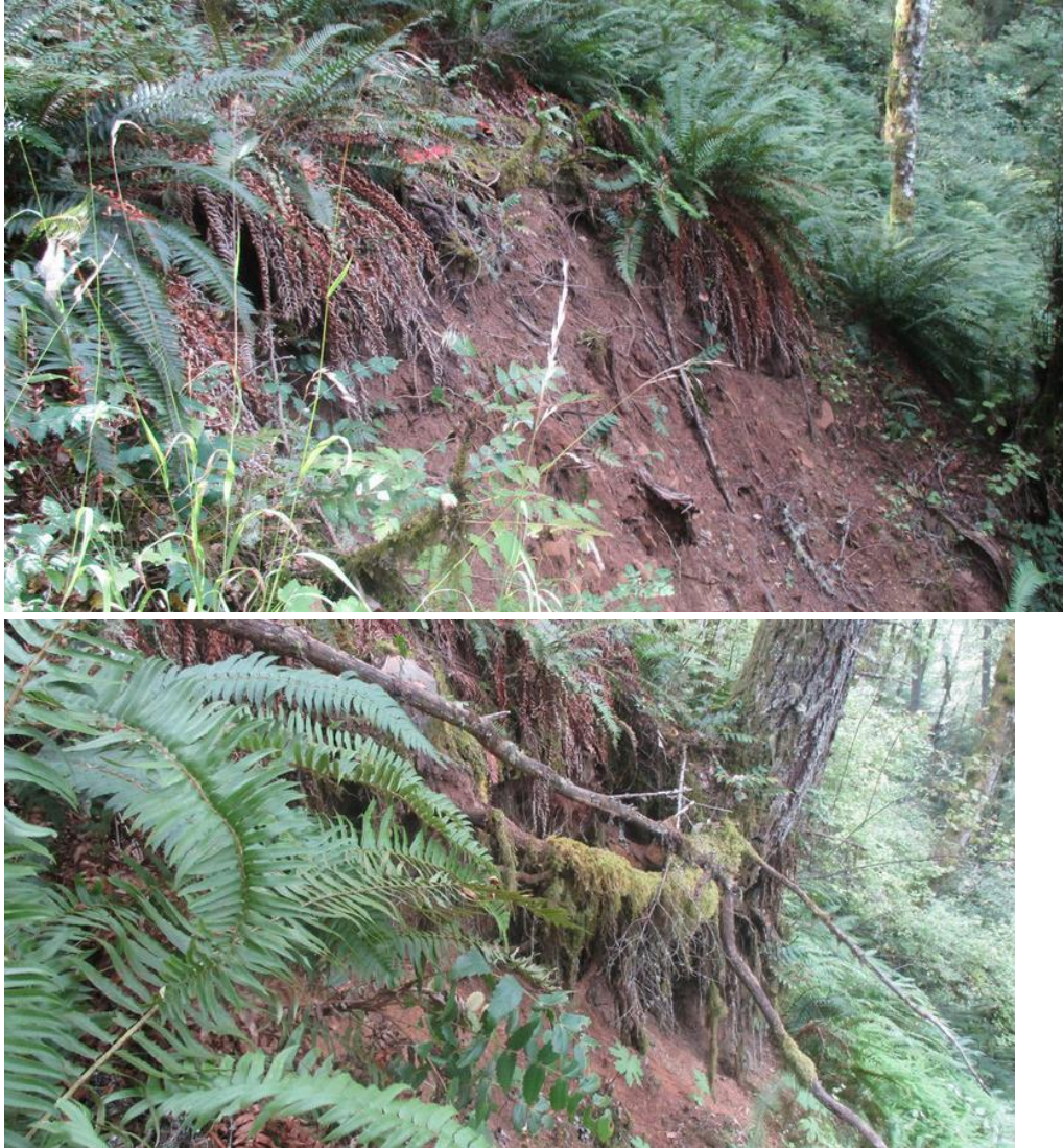
(Above) Landslides within Unit 16
