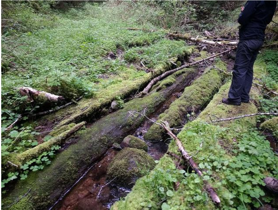
4613-205 crossing of Dry Creek
