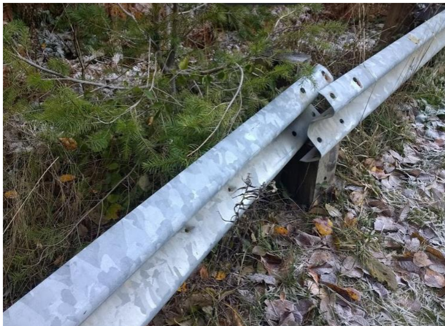
The guardrail (45.20734, -122.14830) at the closed 4613-200 at 4613 (North Fork crossing)
