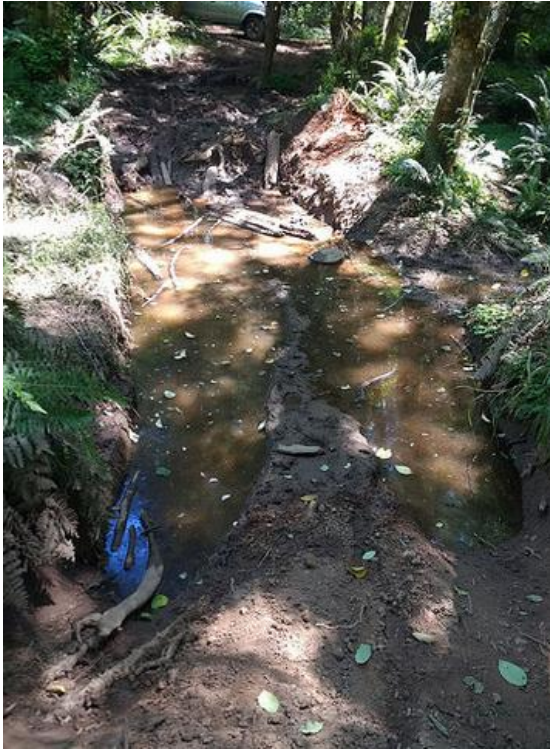
Rd 4614-120 becoming impassible at Unit 148. At the time this photo was taken in summer of 2018, it appeared that several forest users had attempted to breach and circumvent this section of road which evidently acts as a closure
