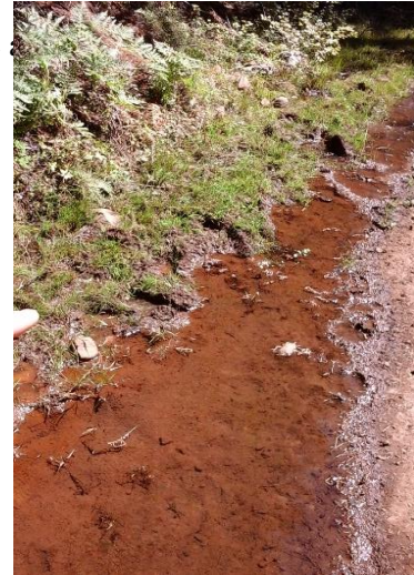
Figure 13. Seep on temporary road on a converted trail surface
