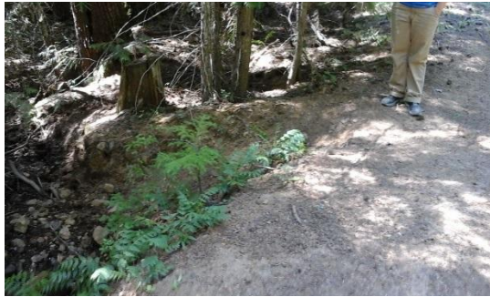
Figure 14. Sediment delivery to a perennial stream channel on a converted trail, temporary road
