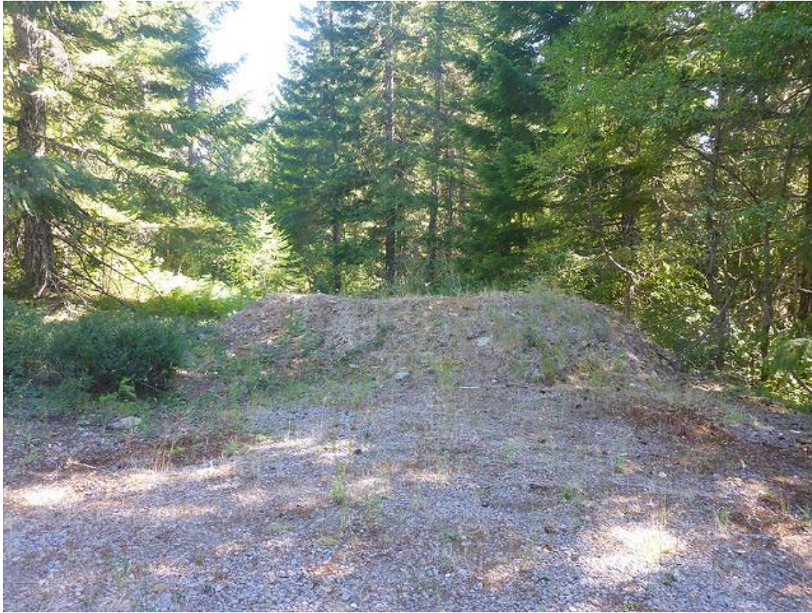
Figure 11: "Decommissioned" FSR 5731-118, with Entrance Management
