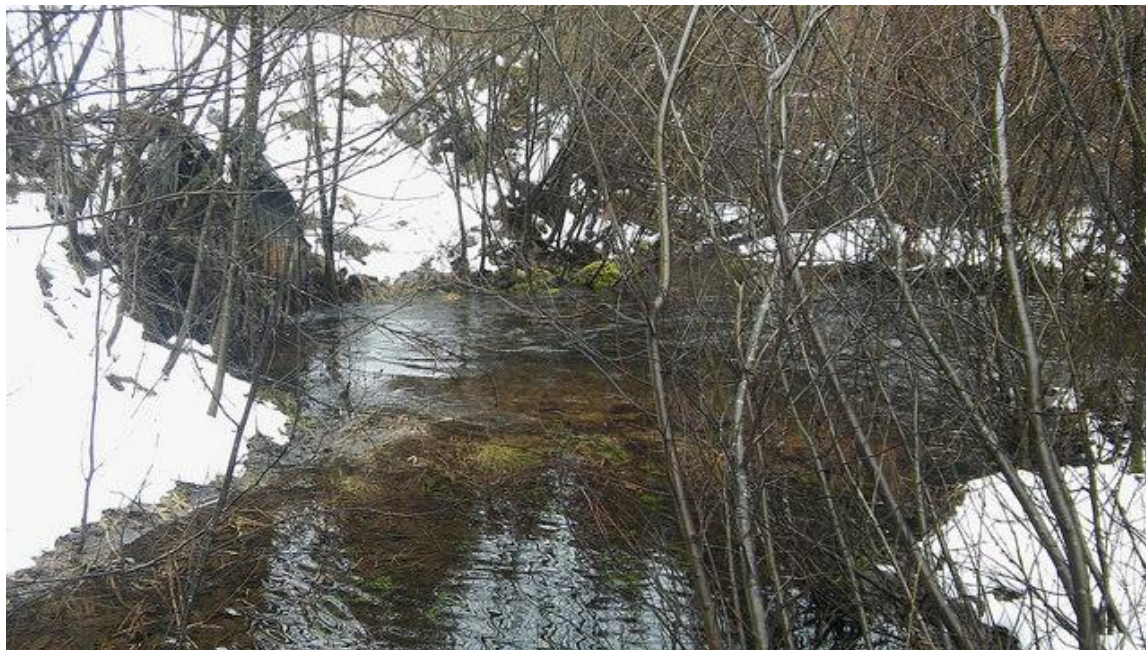
Figure 12: Pot Creek culvert (L) at north side of FSR 46
