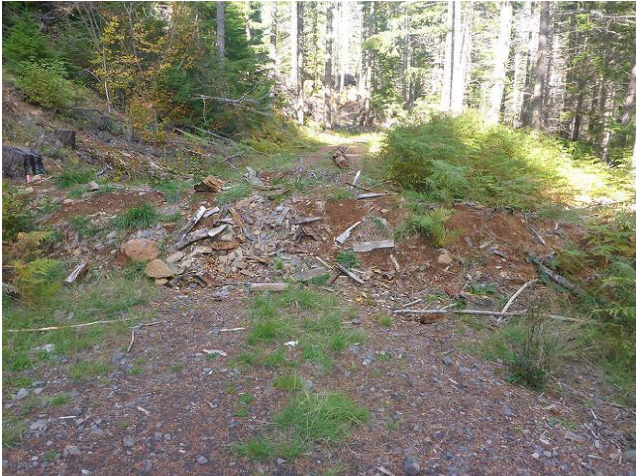
Figure 3: Berm at FSR 4651-140
