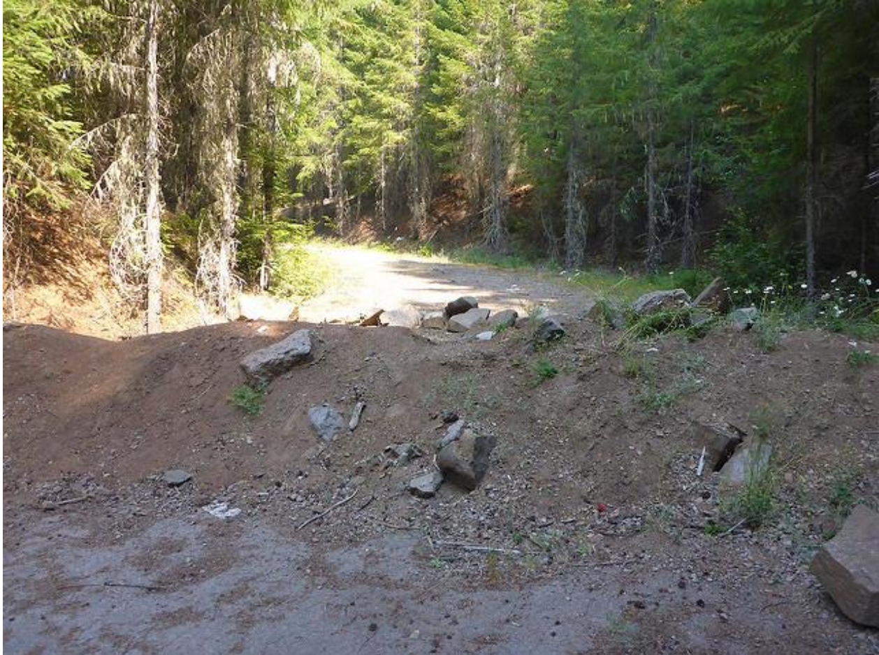
Figure 4: Berm at FSR 4660-120
