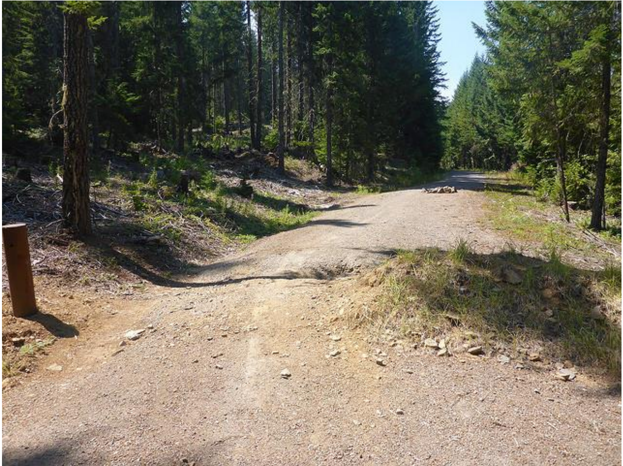
Figure 1: Breached berm at FSR 4660-140
