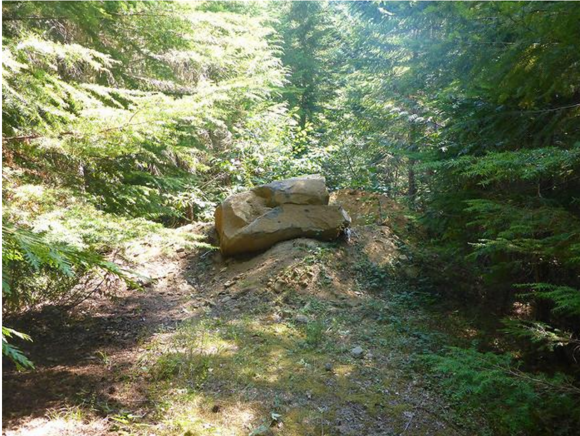
Figure 9: "Closed" road 4661-120, much of which is now passively decommissioned
