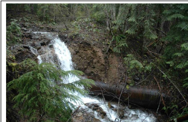
PHOTO 5: Culvert being bypassed on 6322-170.
