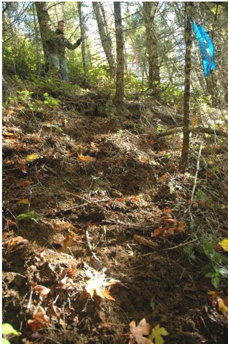
PHOTO 3: Soils on slope below proposed re-opening of road in Unit 3 eroded from footsteps.
